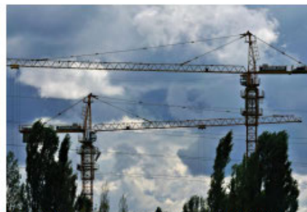
Figure 3: Cranes are especially vulnerable to lightning.
